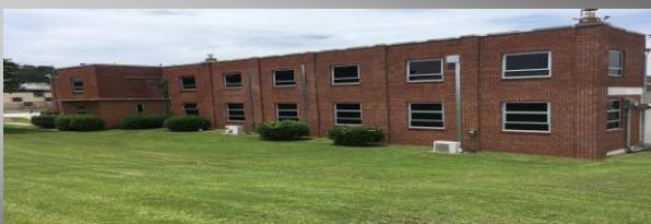
West Columbia Riverside Treatment Plant
