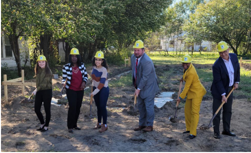
Groundbreaking for new home on Monticello Street Build in South Carolina since 2019.
