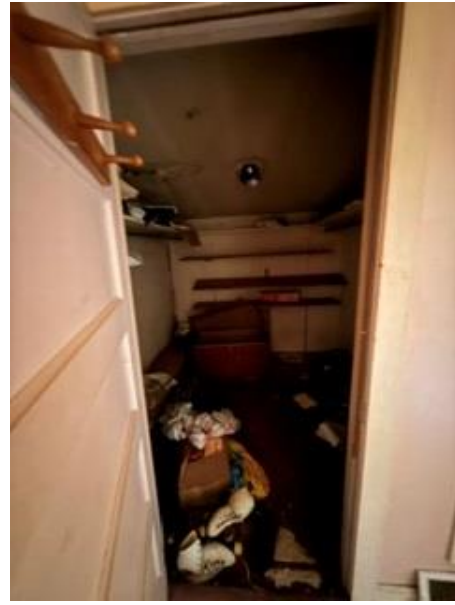
Hallway Closet – texture ceiling (SM2) and sheetrock walls (SM1)
