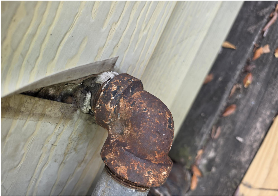
SM9 - pipe caulking 4% asbestos
