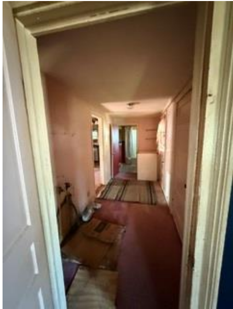
Hallway – texture ceiling (SM5) and sheetrock walls (SM1)
