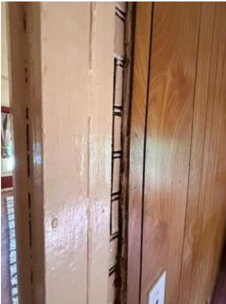
Kitchen Paneling over sheetrock (SM1)
