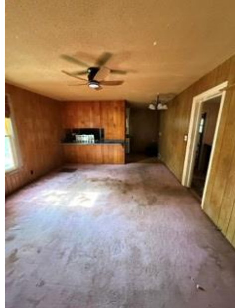
Kitchen - texture ceiling and sheetrock walls
