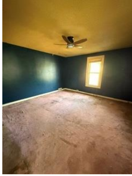
Bedroom – texture ceiling (SM2) and sheetrock walls (SM1)
