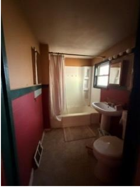
Bathroom - texture ceiling and sheetrock walls
