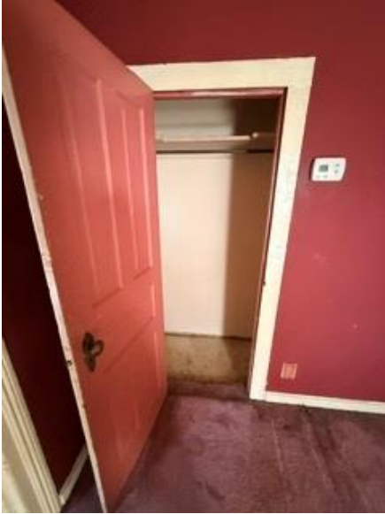
Living Room Closet - texture ceiling and sheetrock walls
